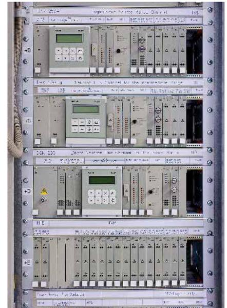
The system proTK covers the requirements for measuring equipment used for the reactor protection system according to IEC61226 Cat A.
