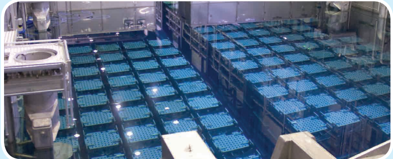
Nuclear facility pool storage
