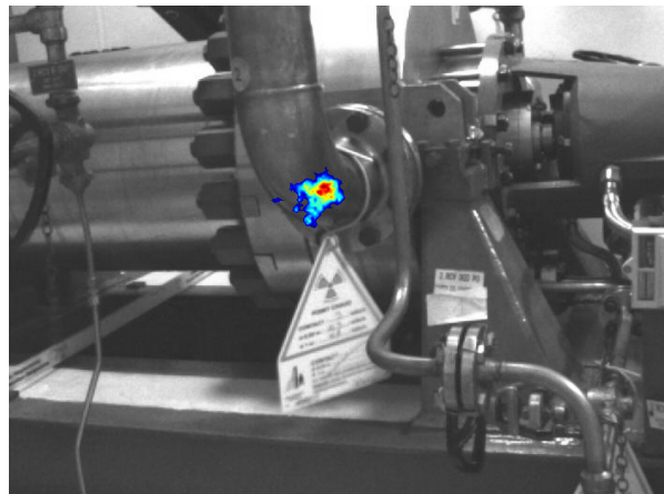
Hot spot detected while surveying piping
