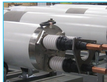
Canister Design, Medium Voltage Power (5kV through 15kV)
