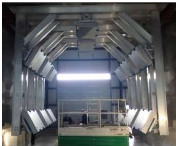
Fig. 6 Installation of the three detector rings within the LINAS chamber.
